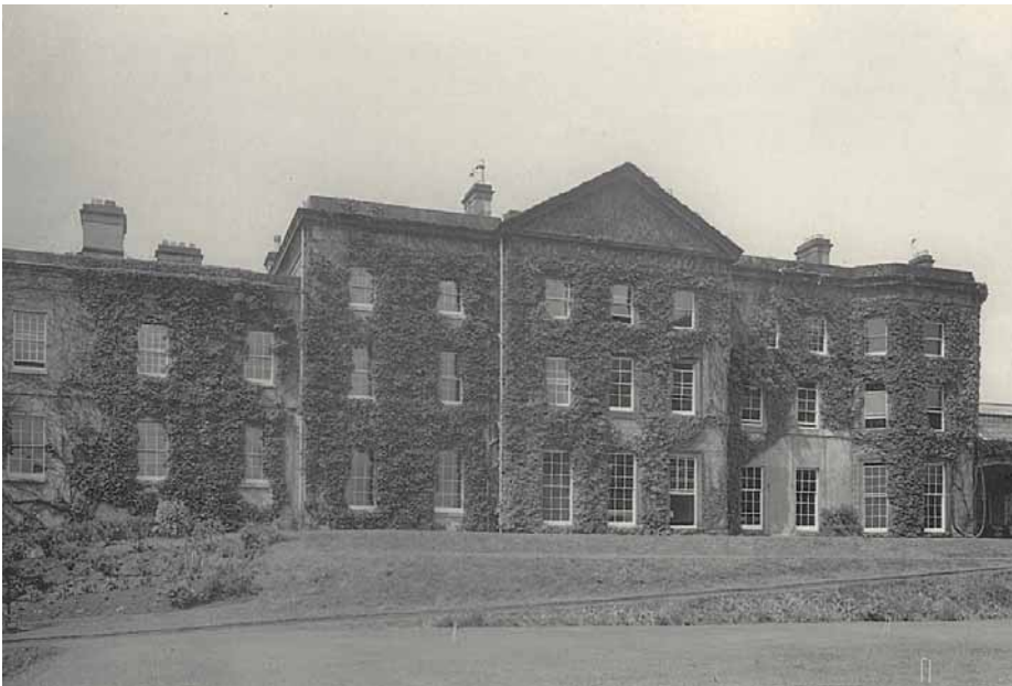
South aspect. The ivy was strong enough to support a climb.
