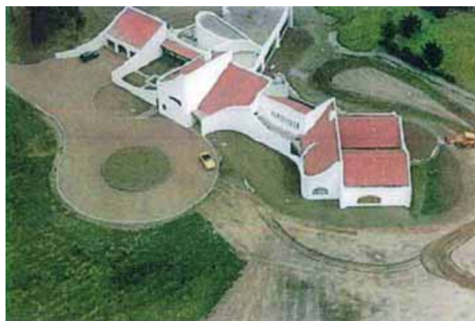
The new house on the site.
