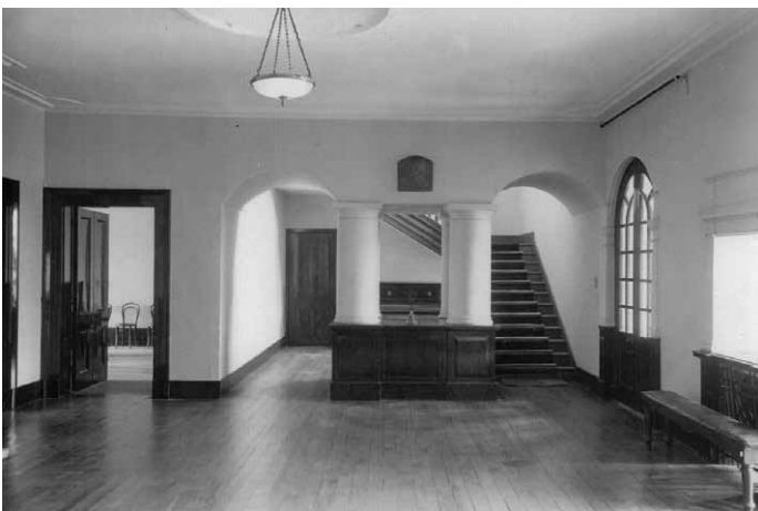
Main hall. Open door into the senior boys refectory. Door to its left into the library.
